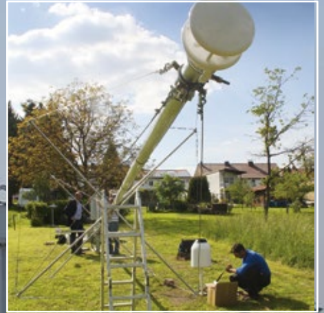
WS sensors have standard interfaces and can be installed at different heights in accordance with WMO requirements.
